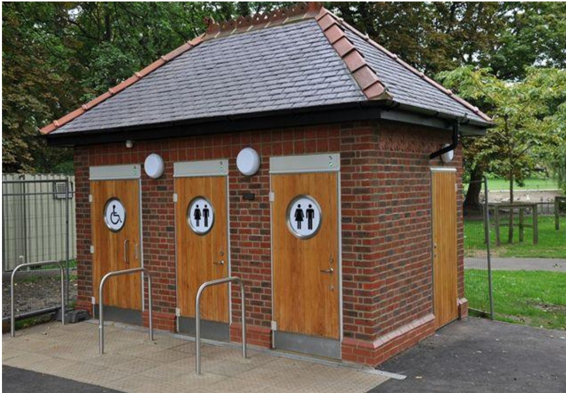
A toilet in England designed by HealthMatic
